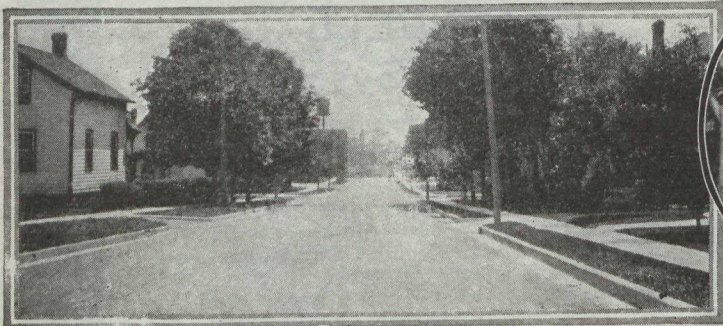
Edwards Street, Kitchener, Ont., "Tarvia-X" pavement.
