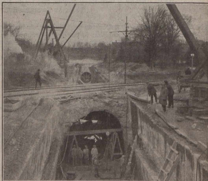
TRENCH FOR WOOD STAVE PIPE THROUGH ROCK SECTION, SHOWING TUNNEL BENEATH INTERNATIONAL RAILWAY CO.'S TRACKS—BOTH SIDES OF CUT ARE CHANNELLED HERE
