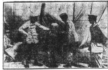
HUNS OVERHAULING A GERMAN "SAUSAGE" Observation balloons, called "sausages," are delicate things to handle, but owing to hard service must often be inspected. Inspection is made of the inside and outside of the envelope. Our photo shows officers and soldiers in the "sausage" inspecting the inside.
