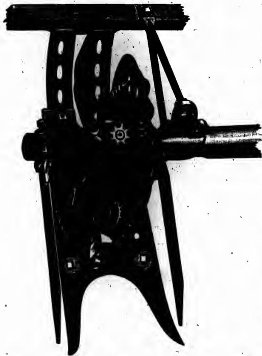
Examine closely the construction of this Knotter. **The knotter is the most important part of a Binder.** An otherwise well constructed Binder with a poor knotter is perfectly useless. Our knotter is very simple; always ties, makes a great saving in twine. Knife cuts but one cord—does not get out of adjustment.
