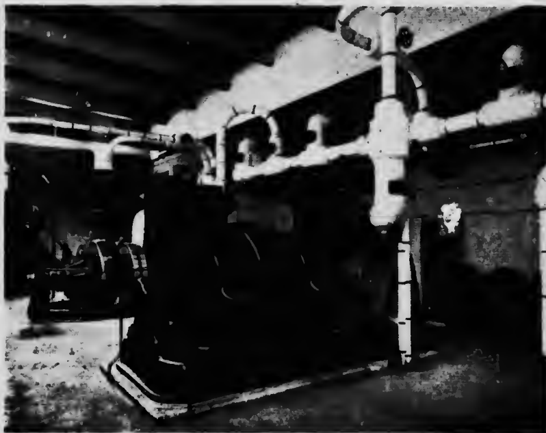
FIG. 2. INTERIOR OF POWER HOUSE ENGINE ROOM SHOWING CURTIS TURBO-GENERATOR IN FOREGROUND WITH ALLEN HIGH-SPEED UNIT IN REAR.
