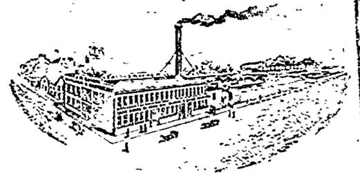
Mr. Eaton operates a large planing mill, which is shown herewith. The factory, which was first erected in 1887, now consists of a two-storey metallic-covered frame building, 60 x 115 ft., with brick engine room and dry kilns. It is fitted with the latest designs of wood-working machinery, and every facility to meet the demands of his extensive trade. The stock rooms are always well filled with finished work. Mr. Eaton has a very commodious and beautifully finished office.
