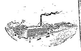
Mr. Eaton operates a large planing mill, which is shown herewith. The factory, which was first erected in 1887, now consists of a two-storey metallic-covered frame building,  $60 \times 115$  ft., with brick engine room and dry kilns. It is fitted with the latest designs of wood-working machinery, and every facility to meet the demands of his extensive trade. The stock rooms are always well filled with finished work. Mr. Eaton has a very commodious and beautifully finished office.
