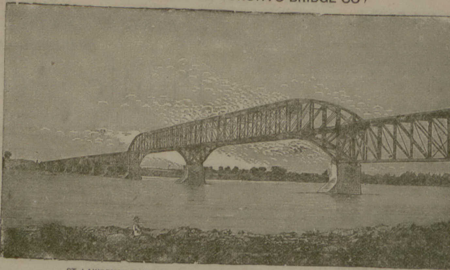
ST. LAWRENCE RIVER BRIDGE, CANADA PACIFIC RAILWAY, LACHINE, P. Q.
