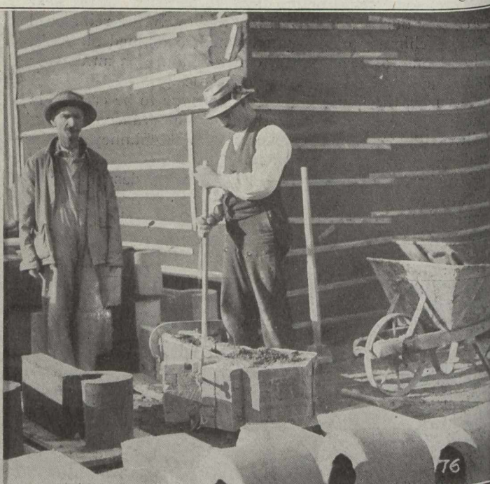
Fig. 10.—Tamping Concrete in the Forms.
