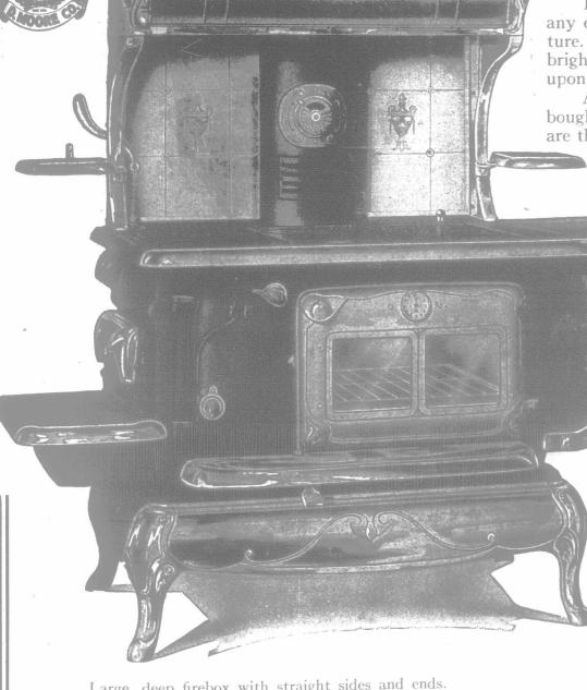
Large, deep firebox with straight sides and ends. Patent Fuel Saver cuts fuel bills in half.
