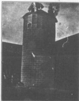
Cement Silo on A. C. Hallman's Farm
