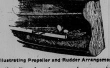
This feature of the propeller being in a tunnel also protects the propeller and rudder both from striking the bottom in shallow places and from tangling in weeds. The accompanying cut will illustrate this
