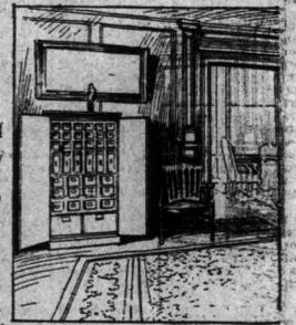
The Globe Steel Safe is built of double walls of cold-rolled steel sheet, insulated both on the outside and inside and with air-tight chambers, making combustion impossible. The case is not soldered or riveted together, but forced together under tremendous pressure. Fitted with Yale key or combination dial lock and made in various sizes. Owing to its light weight, this safe can be rolled on its castors, even the largest size, on any ordinary house floor without damaging carpets or floors.
