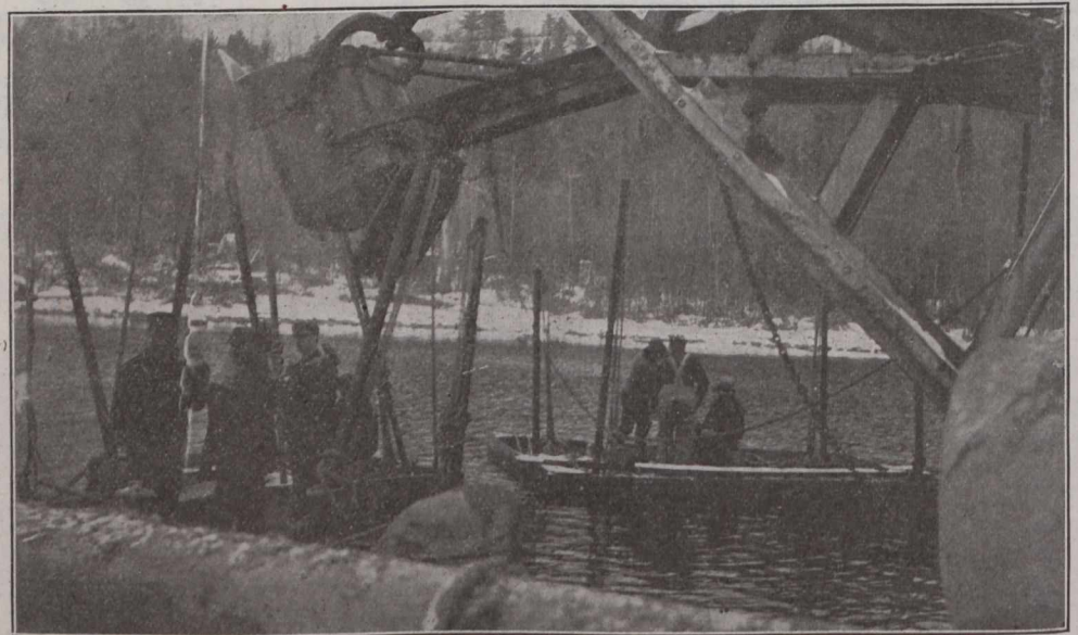
Fig. 5.—Timiskaming Storage Dam, Showing Method of Drilling Boulders Under Water; Dynamite is Loaded into the Drill Hole Through a Gas Pipe, and Exploded by Electric Battery.
