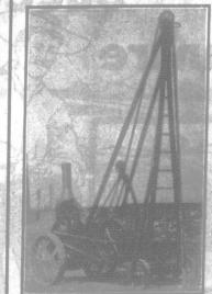
Drilling water wells, or testing mineral land. Run by ateam gasoline or traction engine. Drills wells from two to sixteen inches in diameter.
