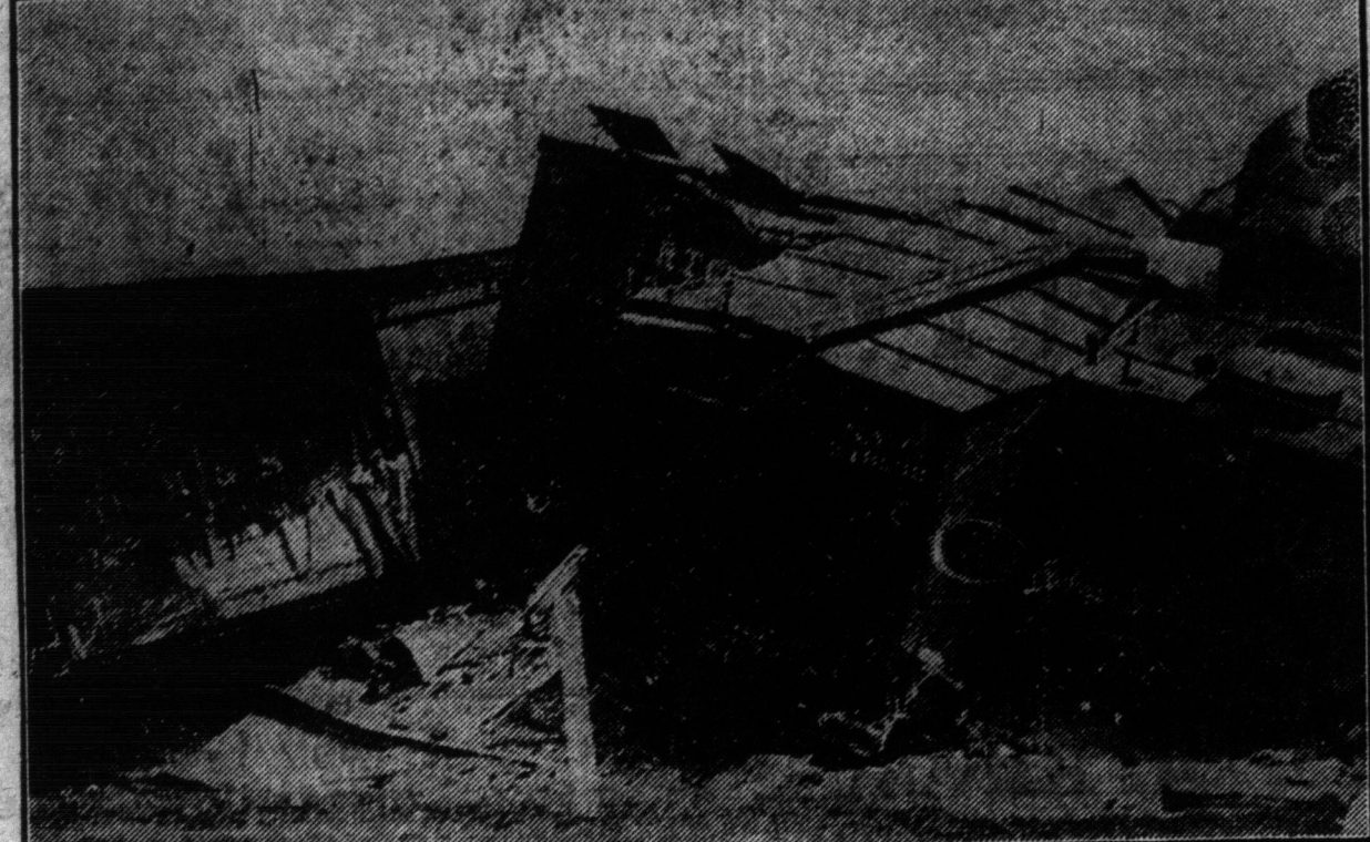
Photograph of part of the wreck of a C. P. R. freight train at Donlands yesterday, when twenty cars were piled up, caused by a spread rail.
