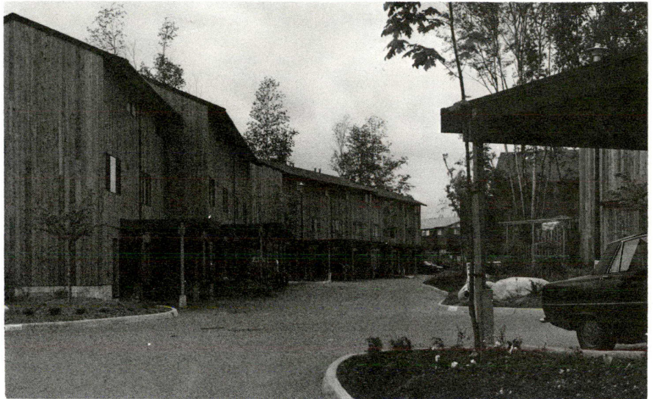
The DeCosmos Village Housing Co-operative, Vancouver, B.C., received the Vincent Massey Award for Excellence in the Urban Environment last
