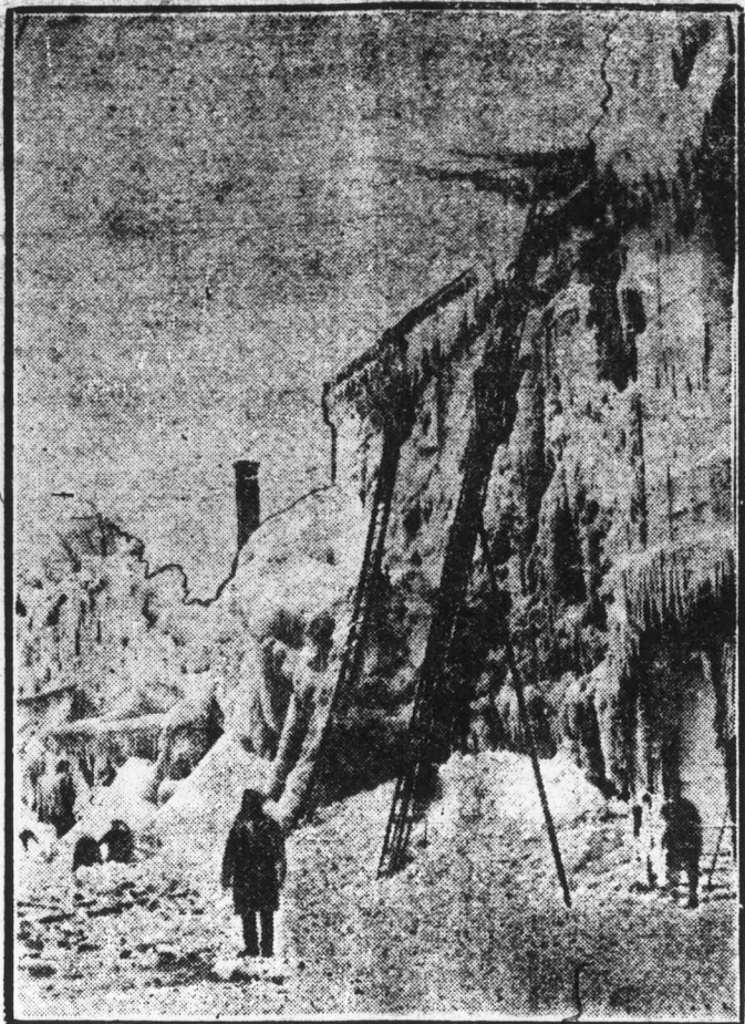
Here is shown the aftermath of a $200,000 fire at St. Hyacinthe, Que., in which the firemen fought the flames in below zero weather, the water freezing shortly after leaving the nozzles.
