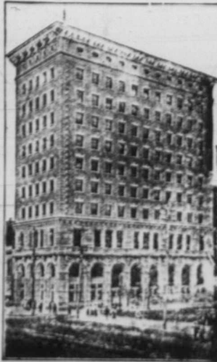
Union Bank Building, Winnipeg
