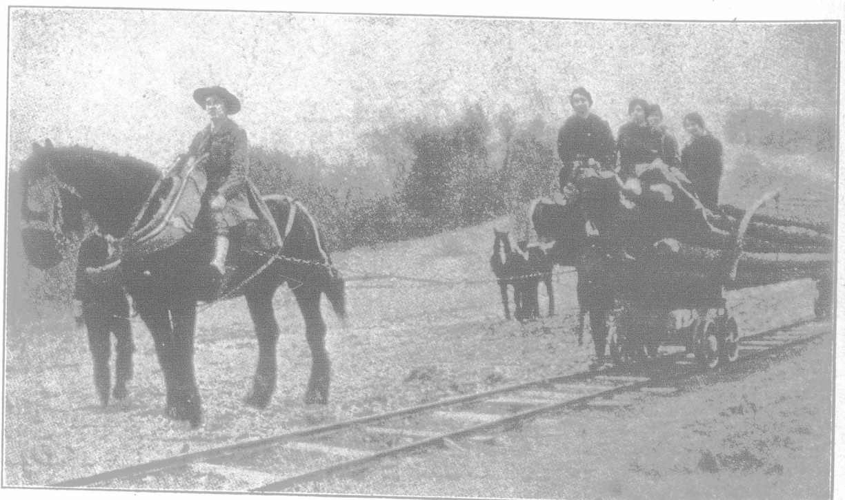
Part of the Timber Corps at Work.
