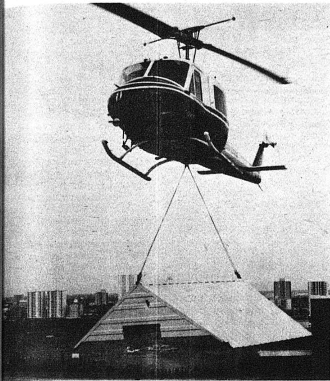
Helicopter installing shelter for Physics building's new acquisition - a telescope. Photo by Robert Smith
