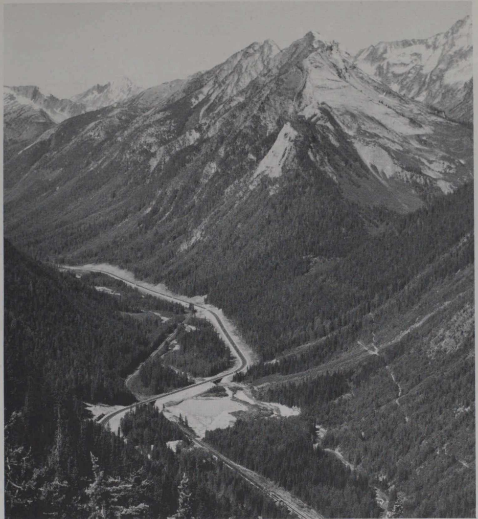
The Rockies are so overwhelming, and the engineering feat of this railway going through them . . .
