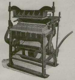
YOJ can use fine gravel and crushed stone with this brick machine as it polishes the face of the brick, and therefore brings the cement to the face of the brick, thus assuring a much stronger brick in the face.
