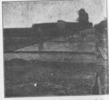
Method of Constructing a Typical Sixteen-Foet Conservet Road The templet used to atrike the crown is shown against the conservet in the for ground. Back of this are the installing devices for a server of balance. They a bolding steel protecting plates in position areas to the conserved before holding steel bardeem Boycod, area are trovelling the surface.
