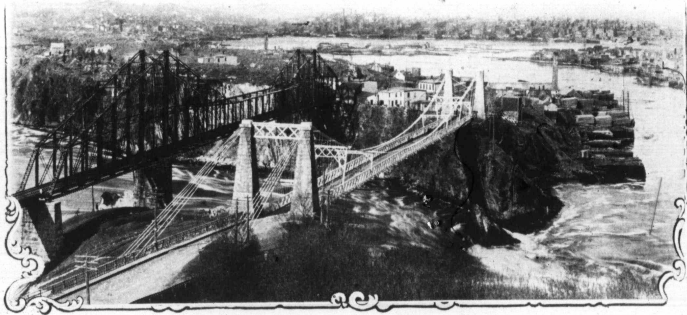
BRIDGES AND FALLS, ST. JOHN, NEW BRUNSWICK.
