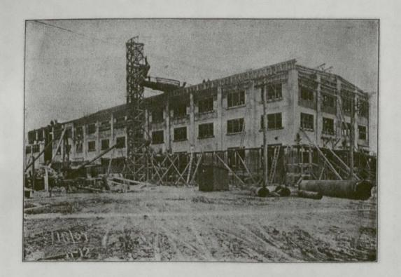
The above picture shows the new works recently constructed of concrete for the Canadian General Electric Company, at Peterborough, Ont. This building from the ground up, as shown, represents thirty-four working days of concreting. The result furnishes an object lesson for speed, economy and excellence of workmanship heretofore unattained in Canada.
