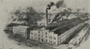
NEW FACTORY BUILT IN 1895 SINCE THEN THE FOLLOWING EXTENSIONS HAVE BEEN MADE MACHINE SHOP LENGTHENED 180 FT. NOW 450 x 120 BOILER SHOP 100 FT. NOW 220 x 80 WITH CORRESPONDING BUILDING SHOP 100 FT. NOW 180 x 80 INCREASE BLACK SMITH SHOP 40 FT. NOW 100 x 40 IN EQUIPMENT.
