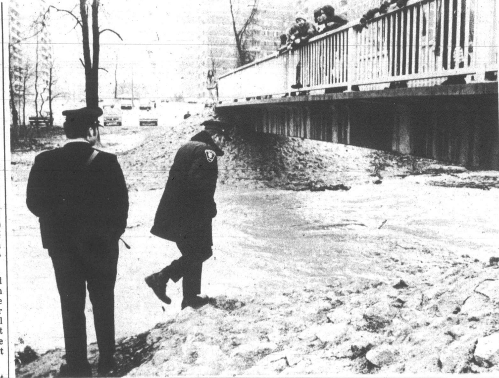
Constables Sean Egan (left) and Tom Kelly inspect a bridge spanning the Cocksville Creek, Mothers in the area say structure is danger to small children because of erosion to its foundation. (See story page 1).
