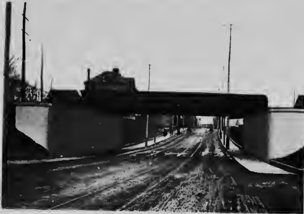
Grand Trunk Bank St. Subway Ottawa.
