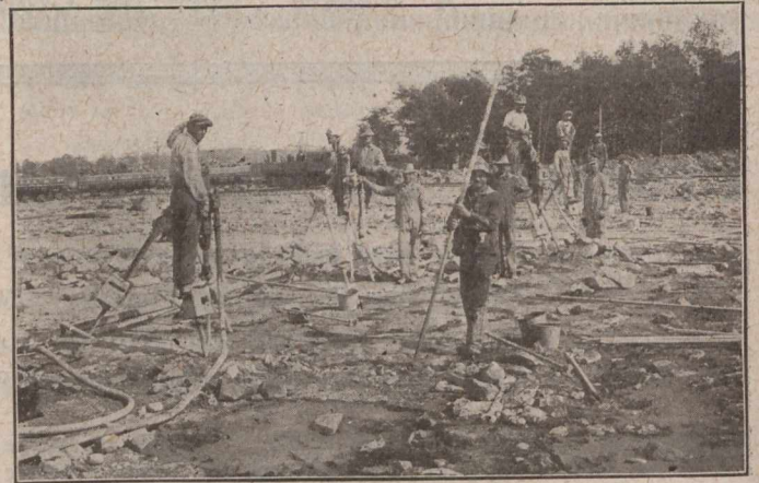
BATTERY OF RAND AND SULLIVAN ROCK DRILLS AT THE FOREBAY
