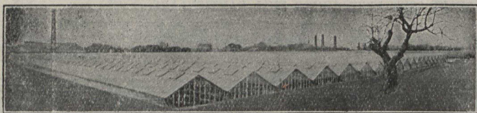
Conservatories of The Dale Estate, Brampton, Ont. Glass supplied by our Toronto Branch
