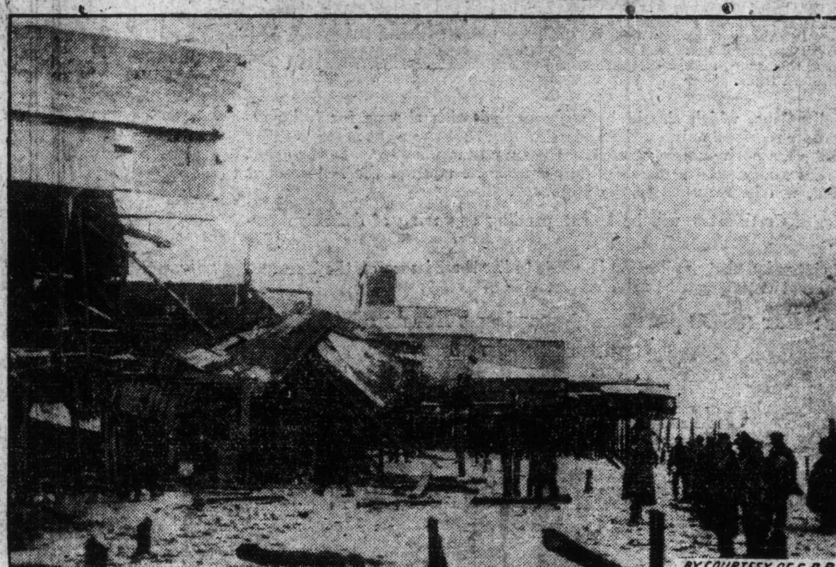
Part of Rockaway Beach, N.Y., after the great storm which smashed four hotels and several iron piers, doing about $2,000,000 damage.
