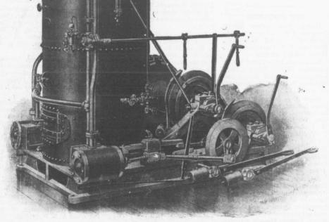
This Double Drum, Double Cylinder Hoisting Engine, a favorite for general contracting work, is one of the different styles we build on "Lidgerwood" designs.
