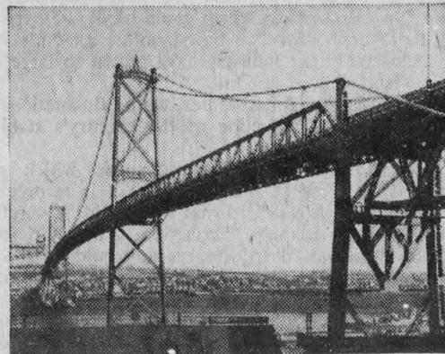
**SUSPENSION BRIDGE IN THE EAST.** The Halifax-Dartmouth bridge, with its main span of 1447 feet and total length of 4420 feet, is the second largest of its type in the Commonwealth—surpassed only by the Lion's Gate bridge, Vancouver, also built by Dominion Bridge.
