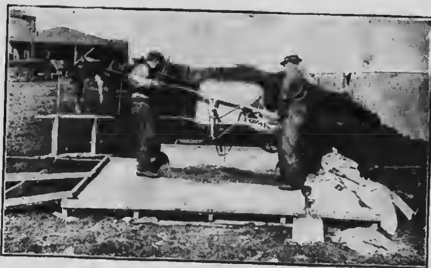
Fig. 8.—Filling the Stone (or Gravel) Measuring Box—First Method.
