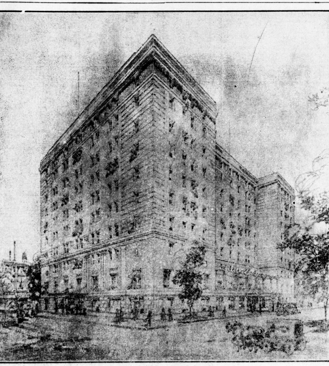
London's long-projected new hotel, to be erected on the corner of Richmond and Pallaton streets, is soon to become a reality. Construction will go ahead in a short time. The Advertiser was told Wednesday.
