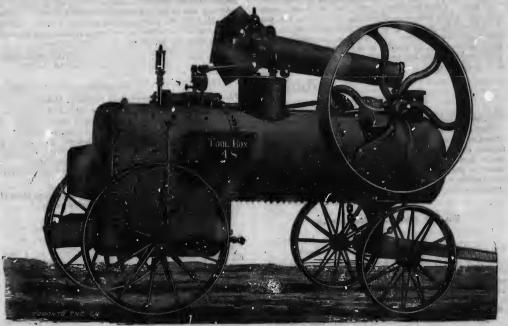
Every Engine Thoroughly Tested with Cold Water and Steam Pressure to 125 lbs, per Square inch.
