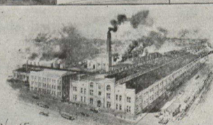
NEW FACTORY BUILT IN 1895 SINCE THEN THE FOLLOWING EXTENSIONS HAVE BEEN MADE MACHINE SHOP LENGTHENED 140'1" NOW 440'4"10" BOILER SHOP 100'1" NOW 220'4"10" WITH CORRESPONDING INCREASE MOULDING SHOP 100'1" NOW 180'4"10" IN EQUIPMENT. BLACK SMITH SHOP 40'1" NOW 100'4"10"
