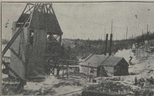
Skip-way, Crusher and Power House
