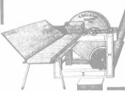
We make the best Ensilage Cutters in Canada whether carrier or blower. Our Exhaust Blower however is, far and away, the best Ensilage Cutter made. The Ensilage from it is thoroughly mixed and pulverized — all hard lumps of ears and stalks are broken up. And it won't choke or clog because the cut corn falls on a shaker chute, which passes it immediately to the blower.
