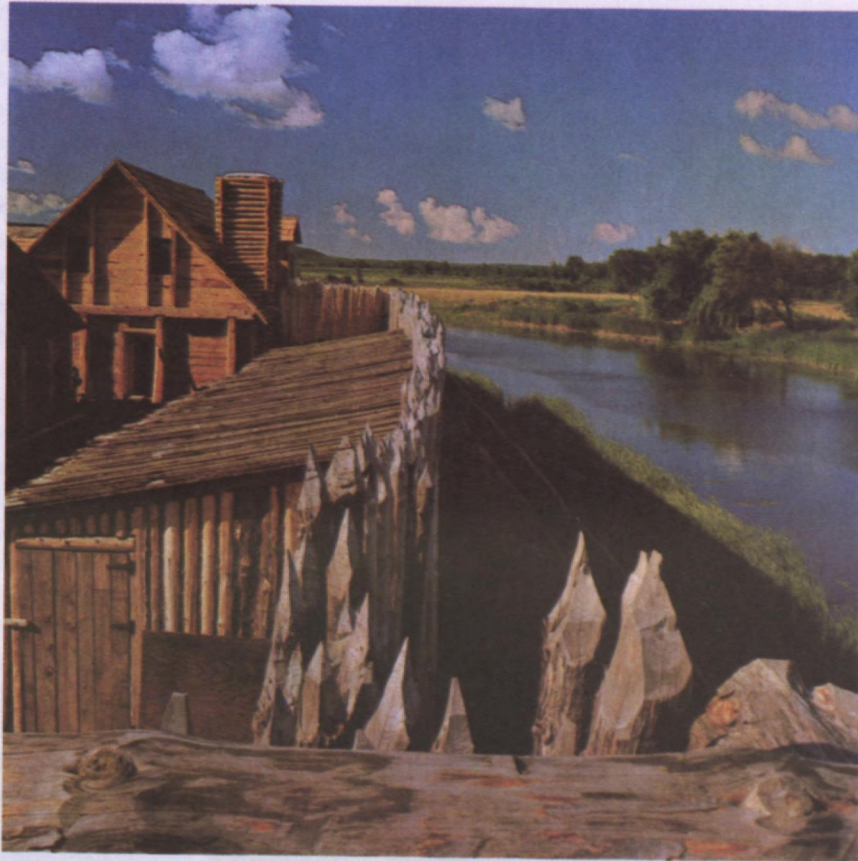
The sharpened logs of its palisade protected Sainte Marie from Iroquois attack
