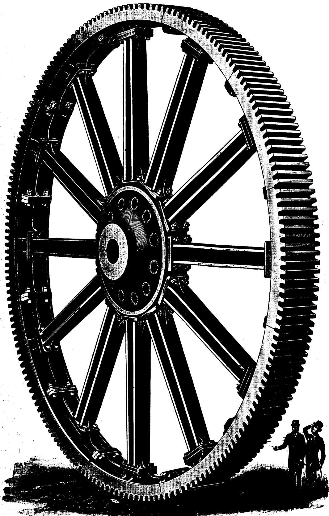
MACHINE CUT SPUR GEAR.
