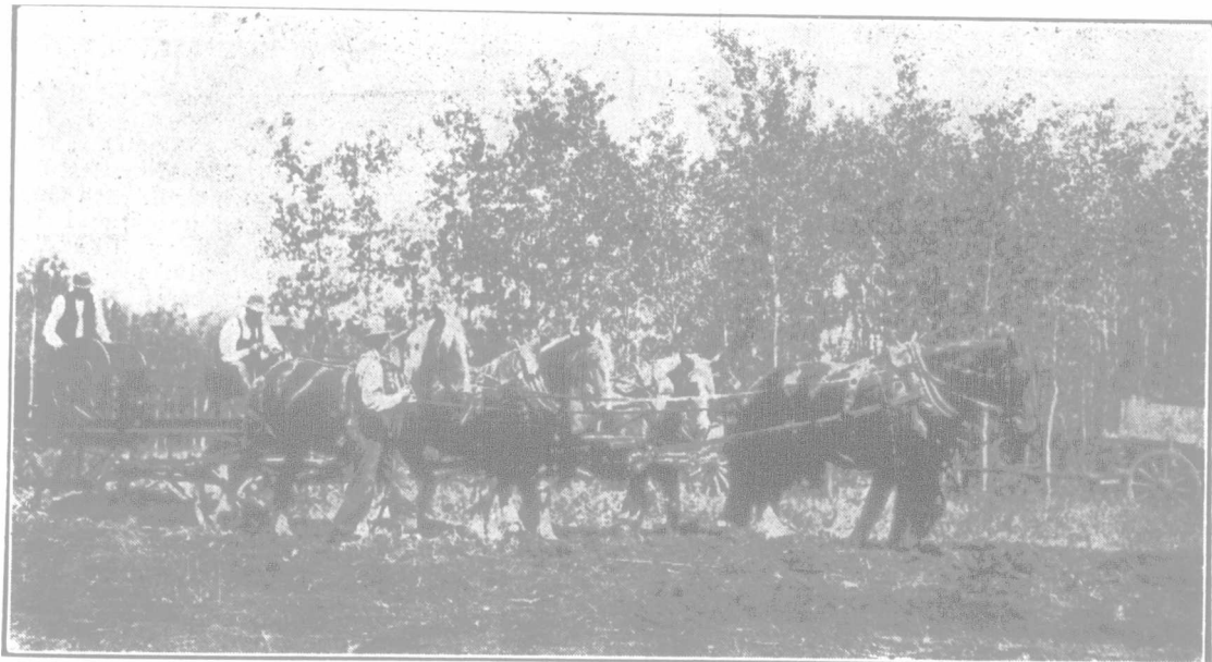
USING THE ROAD GRADER TO MAKE A CROWN AT THE ROAD BUILDING DEMONSTRATION
