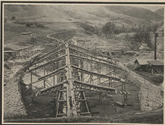
Sluicing an earth dam in Mexico—The earth in solution is discharged through the pipes, and the water runs off leaving the earth behind.
