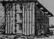
A SIMPLE ICE HOUSE. The cross timbers of the roof are boarded and battened for a roof. Boards are then d over the lower side of these roof timbers, making the roof double, with an open air space between, This keeps off the sun's heat to a very marked degree.
