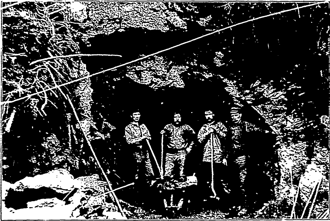
Lower Tunnel, Georgia Mine, B. C.
