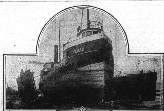
FIRST SHIP TEST OF TORONTO'S NEW DRYDOCK The John Ralph is shown herewith drydocked for repairs in the new drydock of the Toronto Drydock company, in the new ship channel. It is the first of its kind in Toronto, and is built in three each section 65 feet wide. The drydock was brought from Sturgeon Bay, Wis.
