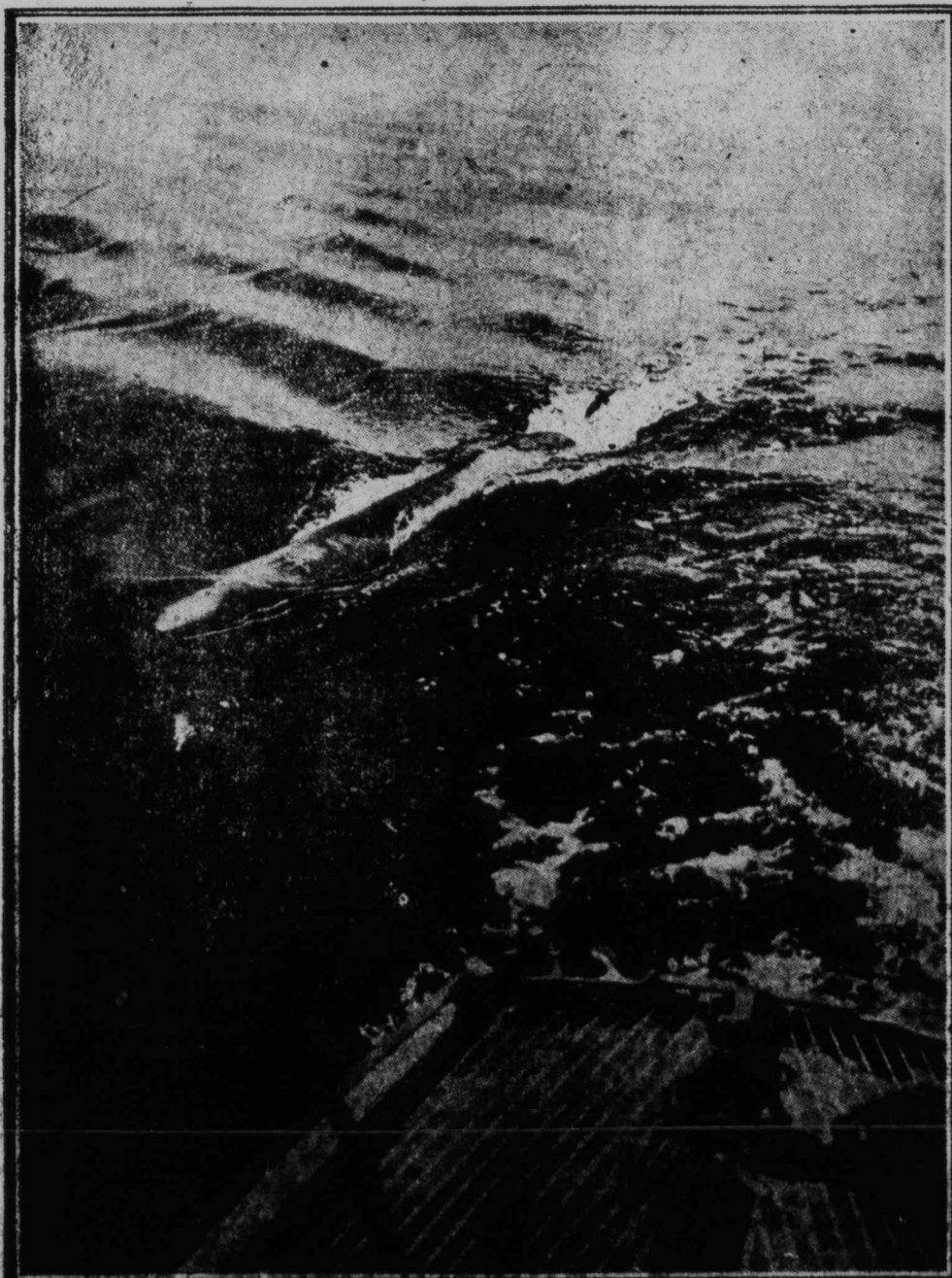
Here is shown an unusual photograph of a torpedo which missed its mark, taken from the stern of the vessel when the weapon of destruction was running on the surface. Usually it runs a few feet below the surface and is only visible by a thin trail of white water behind it. Sometimes in a very heavy sea a torpedo may become visible, but this is very unusual.
