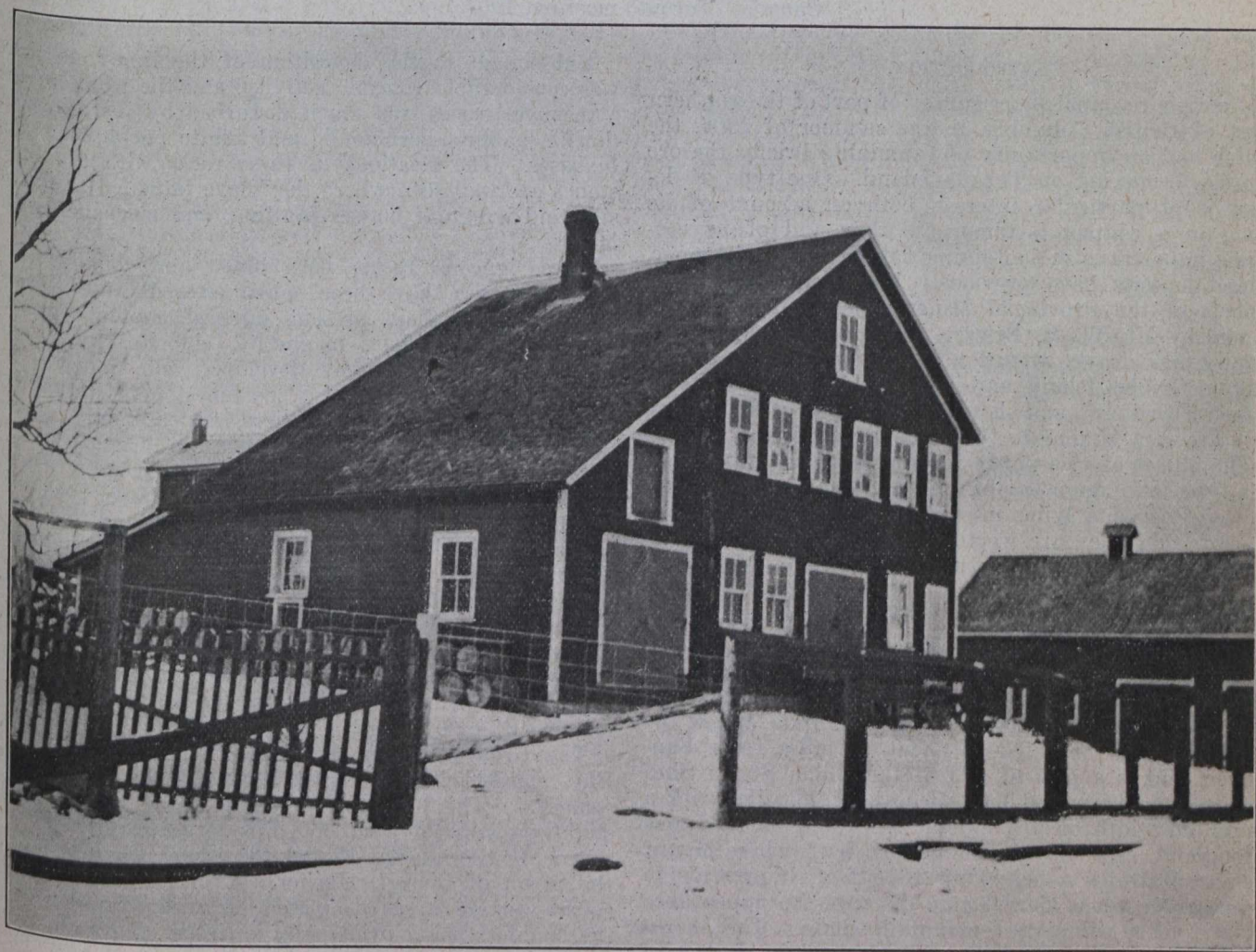
FINISHING HOUSE—LACEY MINE, SYDENHAM.
