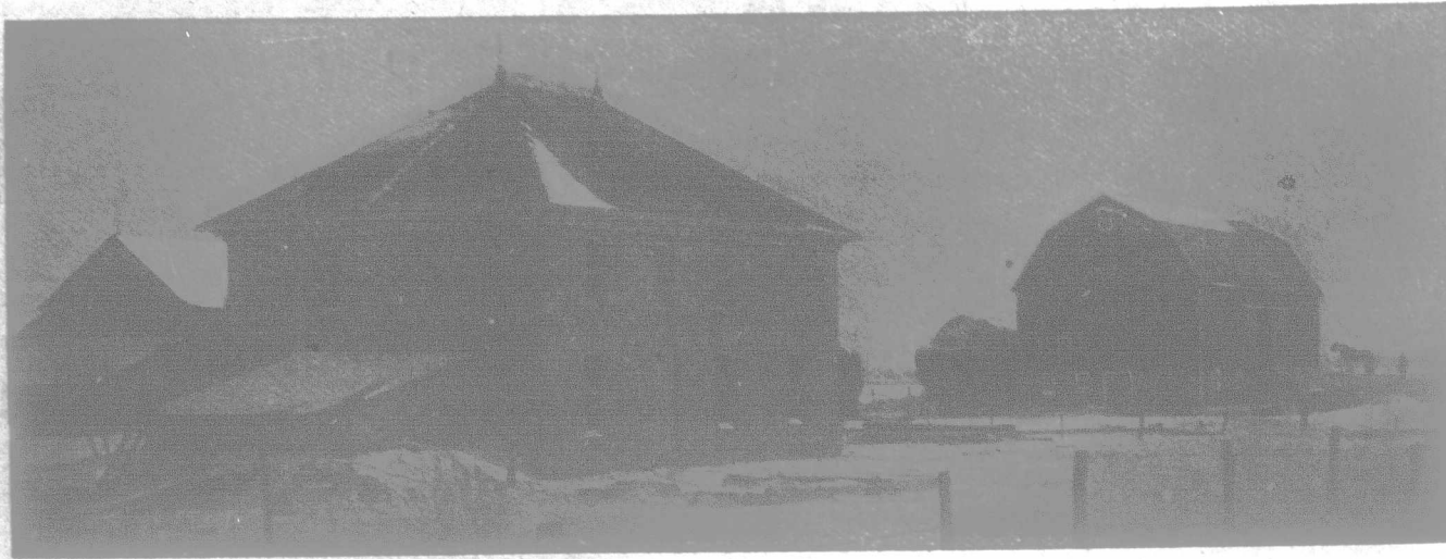
HOUSE AND BARN OF MR. J. E. REAVELY, AT MARSHVILLE, ONT. (Size of house, 28x40x22 high. Size of barn walls, 40x90x10.)
